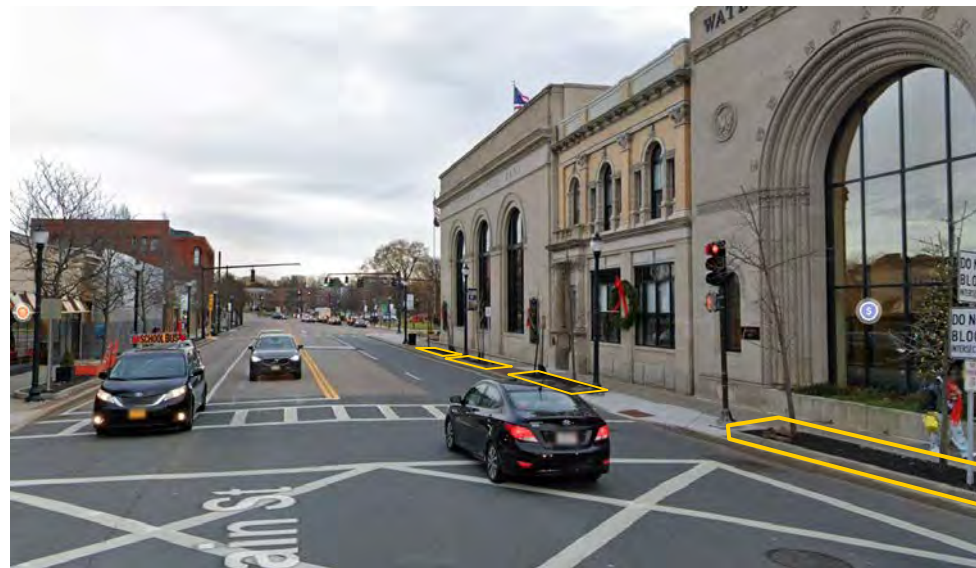
Tree Condition: Critical Main St
