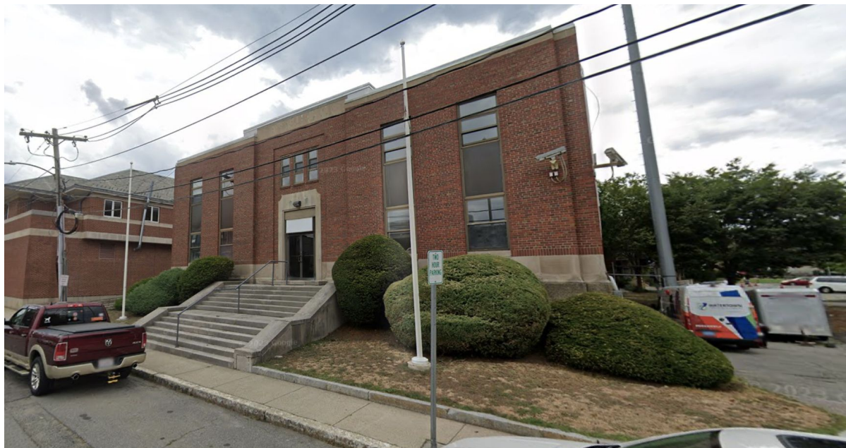
Vacant Police Station
